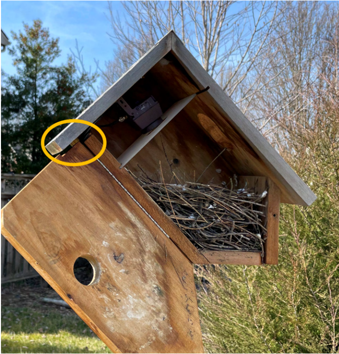
Figure 4. Notches were created at the top of the door and frame to accommodate the installation and removal of the camera and antenna cords.
